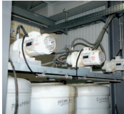
The plastic tanks for storing of the admixtures are filled from level \pm 0 . All fill lines are centrally combined.
